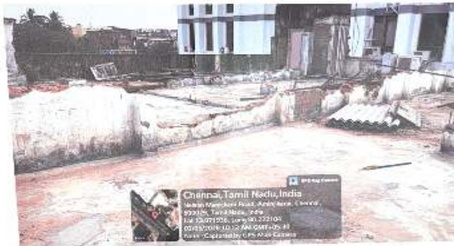
South Side (Front Portion): The Temporary AC Sheet roofing and Brick wall.
