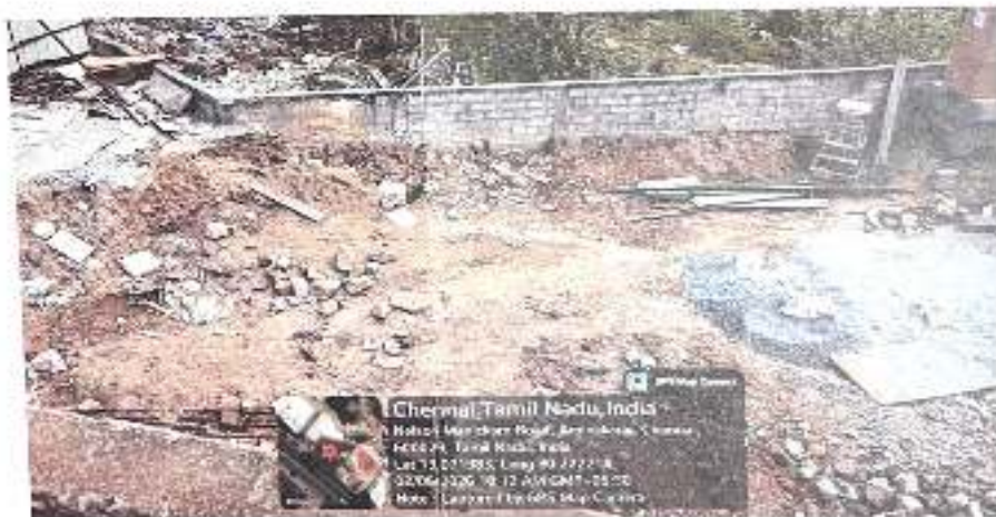
The View of North Side (Rear Portion): Rear Side portion demolished and debris has been completely cleared from the site.
