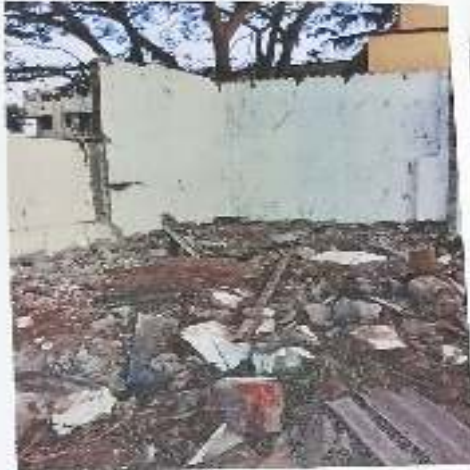
Removal of Shed
