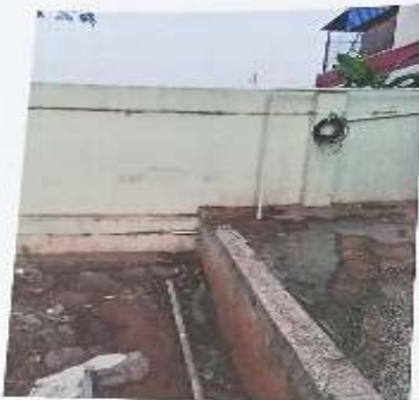
Back End - Water line removed
